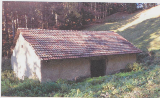
Figure 9 7-07 Rond-Bouéchet, construction massive en pierre naturelle. (Photo N. Gogniat, 2015)
