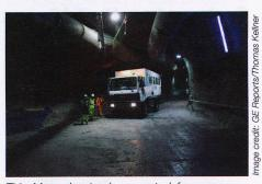
This Mercedes truck converted for passenger travel shuttles through a 3-kilometer-long tunnel (nearly 2 miles) built some 1,800 meters (5,900 feet) above sea level between the cable car and the power plant.
