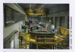
The a so-called pumped-storage power plant generates or stores electricity by moving water between two mountain lakes separated by a 630-meter cliff.
