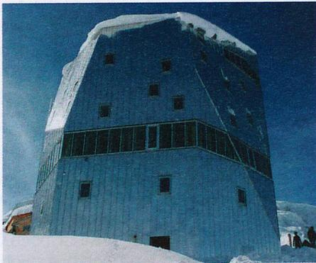
The Monte Rosa hut, a mountain refuge built in 2009 amid high-altitude crags, is in the words of ETH Zurich team that designed it, "Switzerland's most complex wooden building". The hut has stainless-steel foundations, an aluminum outer shell and a computer-controlled energy-management system that employs the same solar panels as the Solar Impulse. Simply put, this is a mountain refuge on the cutting-edge of sustainable development technology.
