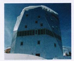
The Monte Rosa hut, a mountain refuge built in 2009 amid high-altitude crags, is in the words of ETH Zurich team that designed it, "Switzerland's most complex wooden building". The hut has stainless-steel foundations, an aluminum outer shell and a computercontrolled energy-management system that employs the same solar panels as the Solar Impulse. Simply put, this is a mountain refuge on the cutting-edge of sustainable development technology. Monte Rosa hut. By Hwking via Wikimedia Commons
