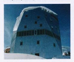
The Monte Rosa hut, a mountain refuge built in 2009 amid high-altitude crags, is in the words of ETH Zurich team that designed it, "Switzerland's most complex wooden building". The hut has stainless-steel foundations, an aluminum outer shell and a computer-controlled energy-management system that employs the same solar panels as the Solar Impulse. Simply put, this is a mountain refuge on the cutting-edge of sustainable development technology.
