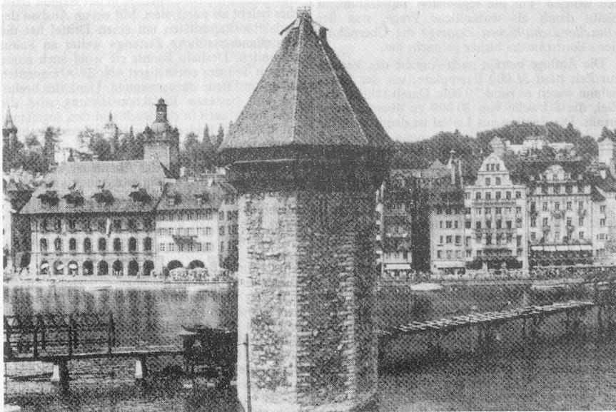
The picture shows what was left of the bridge after the disastrous fire of August 1993. The restoration of the bridge to its original state will have cost over 3.3 million SFR. The wooden construction has been re-built in timber taken from the local pine forests around Lucerne and match as best as possible both ends of the bridge which were saved from the fire. The cause of the fire has still not been fully established.
