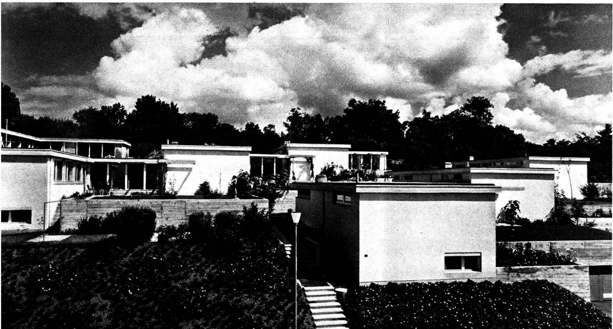
Architectes Danzeisen + Voser FAS-SIA, Saint-Gall
