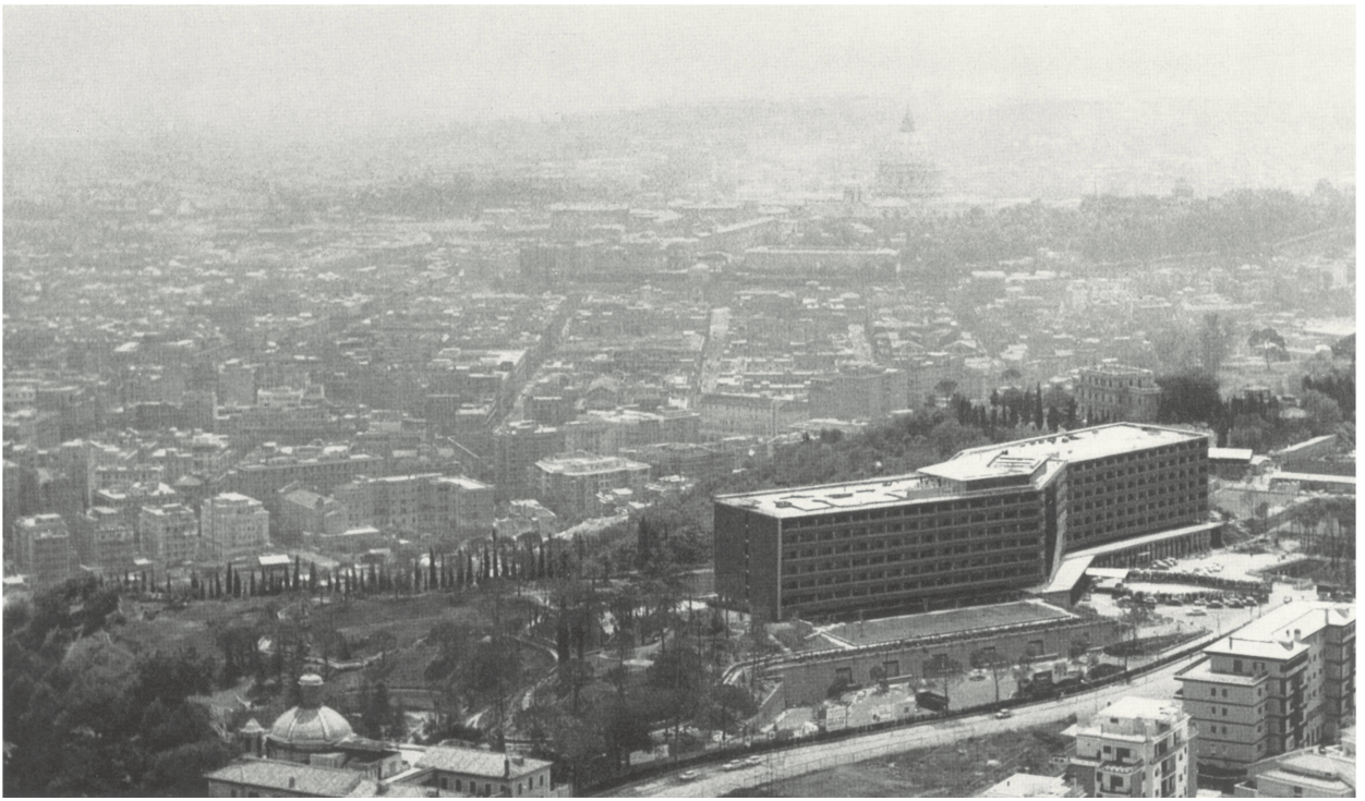
fig. 1 Ugo Luccichenti, Emilio Piffari, and Alberto Ressa, Hotel Cavalieri Hilton (1961–1963), Rome. Source: Vitrum 141, (Jan.–Feb. 1964), 27.
