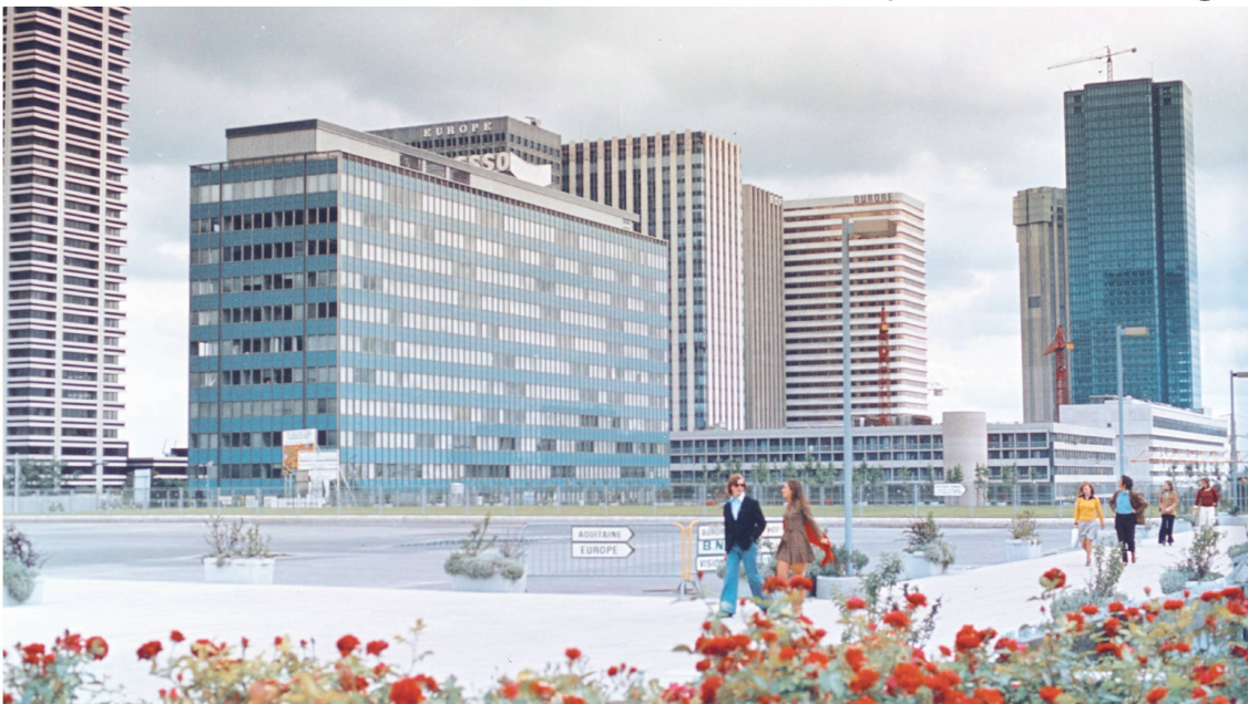
fig.1 Immeuble Esso, designed by Jacques Gréber, built from 1958 to 1963 as the first office building at La Défense. In its early years, varying positions of blinds proudly display the corporate name while flaunting the translucency of the curtain wall, the first in France on this scale. Source: Archives Defacto/La Défense.
