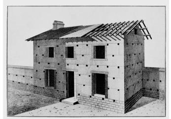
THE ORIGINS OF MODERN CONCRETE 1. The Technique of Pisé Construction (From Rondelet: Traité de l'Art de Bâtir (1812), Vol. I, article 12, Plates V and VI)
