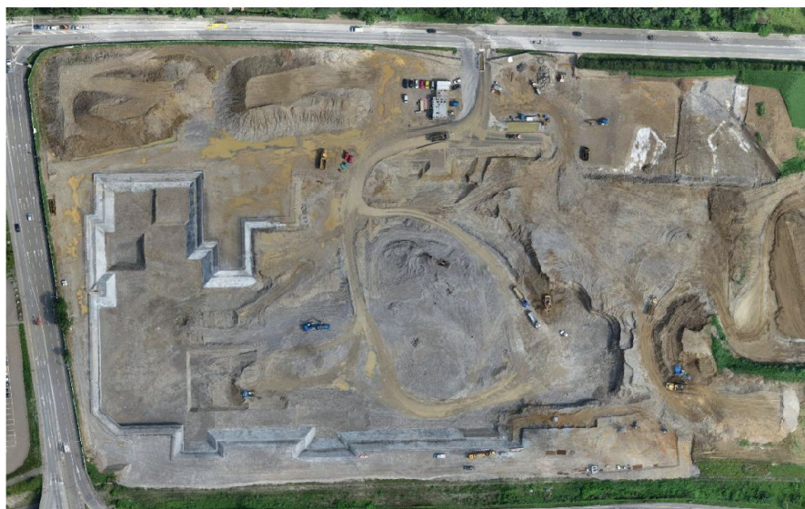
Abb. 1: Aushub. Fig. 1: Excavation. Fig. 1: Scavi.
