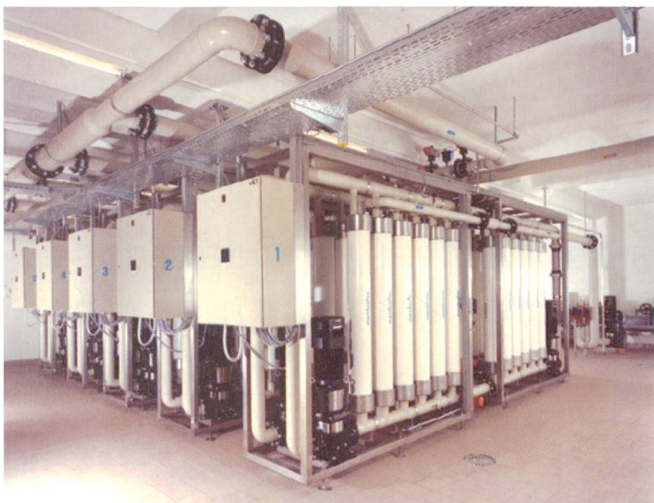
UF-Anlage Lens/Crans-Montana, 450 m 3 /h.
