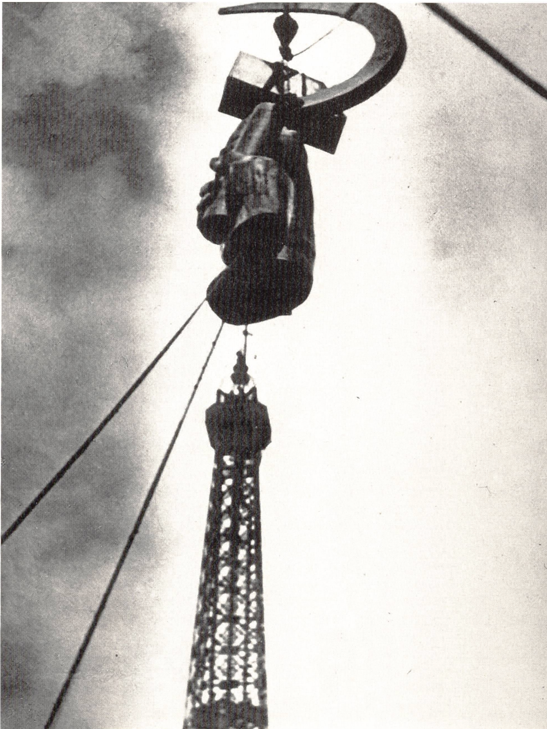
fig. 6: Vera Mukhina, "Industrial Worker and Kolkhoz Farm Woman", Photo of hands hoisted into place, 1937. Two powerful cranes hoisted the pair of hands holding hammer and sickle up and positioned it to be welded onto Vera Mukhina's giant steel sculpture atop the Soviet Pavilion at the Paris World Exposition. A long-exposure photograph was taken at exactly the moment when the Soviet emblem appears to soar over the Eiffel Tower in the far background. The accompanying propaganda literature about the making of the separate parts at a Moscow steel plant and their subsequent assembly on site extols the sculpture as a product of heavy industry and as the collective achievement of artists, engineers, and specialists. Its timely completion redeemed the convergence of art and technology, the theme of the Paris World Exposition, more spectacularly than any contribution from another state.
