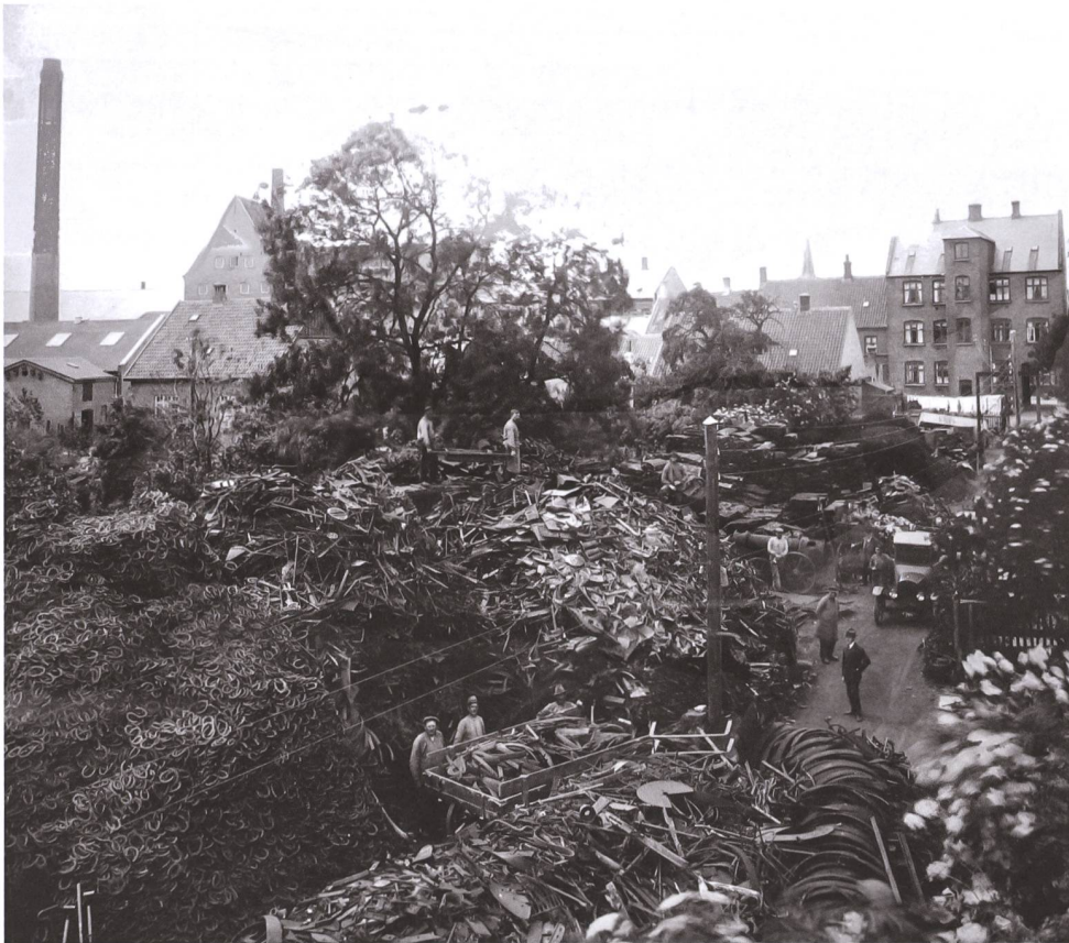
4 The yard of one of Denmark's largest scrap companies in the mid-1920s. Even then, the scrap had to be sorted carefully. For example, the pile on the left consists exclusively of horseshoes.
