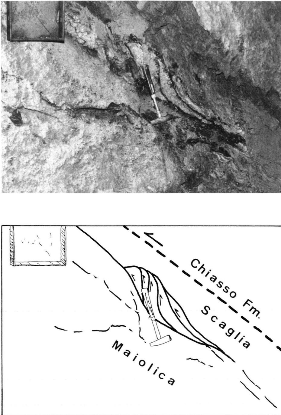
Fig. 4. Photograph and interpretative sketch of the tectonic contact between Maiolica and Chiasso Formation in the new Monteolimpino tunnel. Note imbrication structures indicating a thrust of the hanging wall (Chiasso Formation) from the right (South) to the left (North).
