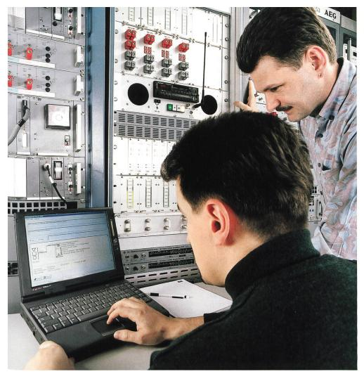
protection and back up, an ISDN link is provided for every main program and can be activated from the studio or the SBC Dist. In the SBC Dist the data are extracted from the MPEG-stream and prepared to be multiplexed into timeslot 16 of the G.703 2 Mbit/s datastream.
