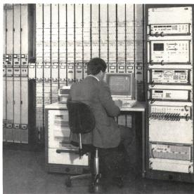
Measuring systems designed for telecommunications applications. These include a data line test system used by the German Federal Postal Authority, an automated monitoring system for the Pacific Submarine cable system, ANZCAN, and automatic line-up measurements via satellite between two earth stations.
