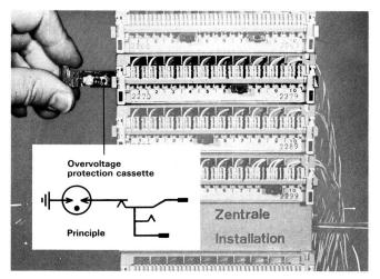
Fig. 11 Overvoltage protection cassette
