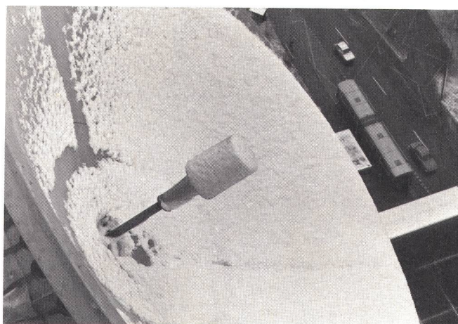
Fig. 9 Snow covered receiving antenna, view from above
