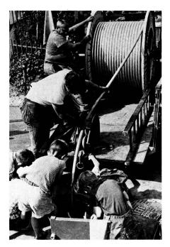
Pose d'un câble coaxial - Laying of a coaxial cable
