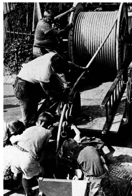
Pose d'un câble coaxial — Laying of a coaxial cable
