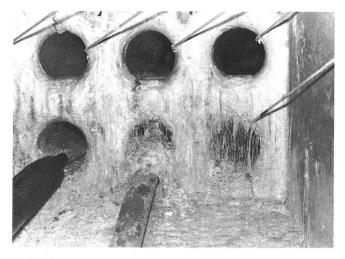
Fig. 5 Multiway duct at Arbon, fault site
