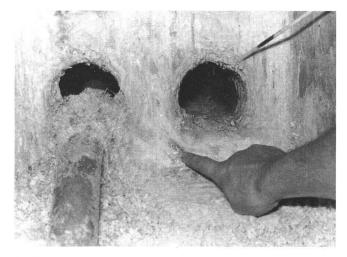
Fig. 6 Multiway duct at Arbon, fault site
