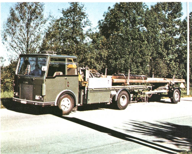
Stangentransport Transport de poteaux Pole transport
