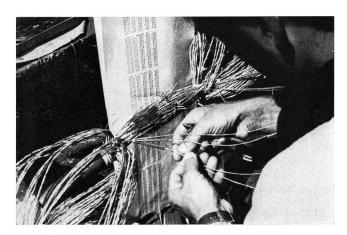
Splicing of a star-quad telephone cable with the aid of a computercalculated table
