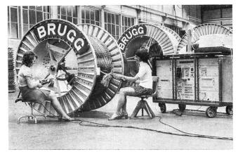
Operators testing a factory length of cable by means of automatic tester KMA-3b
