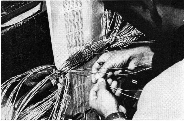
Fig. 7 Splicing of a star-quad telephone cable with the aid of a computer-calculated table
