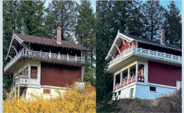
The Edward Feuz Chalet: Before and after exterior renovations. Photo credit: Montayne
