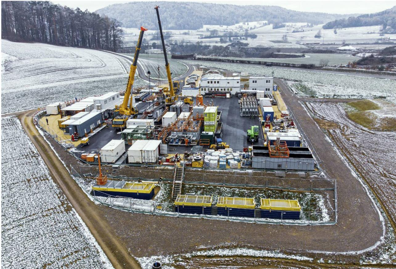
Nagra has carried out test drilling, such as here in the vicinity of Stadel, into the deep layers of underground rock. The magic ingredient is Opalinus. It is currently believed to be suitable for storing radioactive waste.
