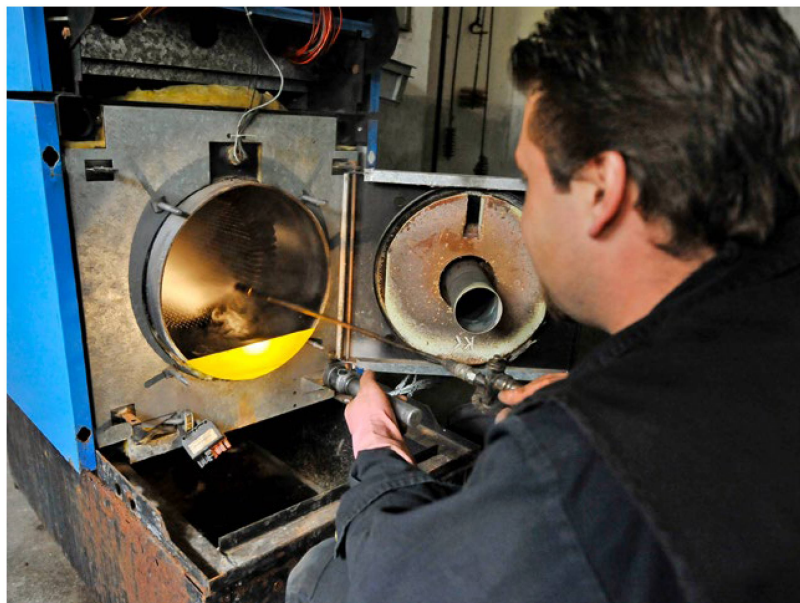
A chimney sweep cleans an oil furnace and has many more to do. Although they are growing obsolete, a surprising number of new oil heating systems are being installed. Photo: Keystone
