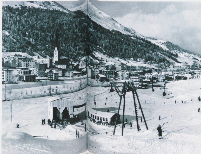
The "Bolgenlift" in Davos was the world's first t-bar ski lift, photo from winter 1934/35
