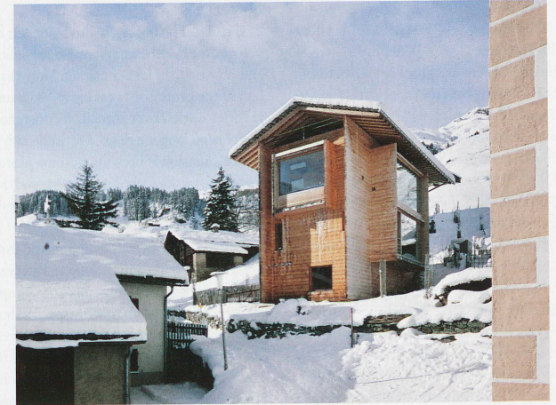
A house built by the architect Peter Zumthor in Leis photographed by Ralph Feiner in 2012
