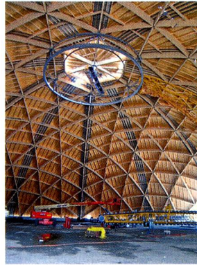
Riburg 2005: Rheinsalinen's logistics and storage centre with a 31-metre-high wooden dome
