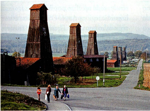
Zurzach 1978: The wooden pumping towers above the Sodafabrik's drill holes sunk in 1914 are listed as an historical heritage site
