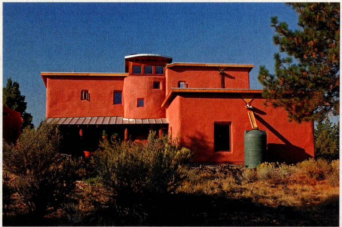
The small windows on the North side of the house minimize heat loss. Rainwater run-off from the roof is collected for re-use.
