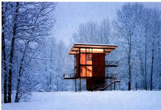
The three-story steel cabin on stilts in Mazama, Washington, that can be completely shuttered with the turn of a hand crank
