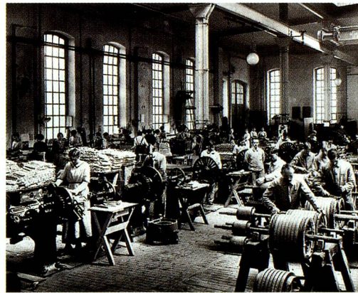
The BBC factory in Münchenstein (1915). Manufacture of magnetic coils for use in locomotive engines.
