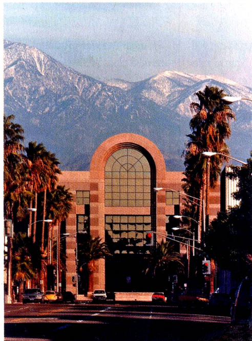
San Bernardino County Government building
