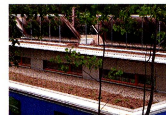
Extensive green roof of Waldsee BioHaus that serves to retain rainwater, reduce the risk of erosion and act as a heat buffer during the summer.
