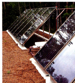
Solar panels which are part of a sophisticated solar hot-water system that meets the high volume hot-water needs of Waldsee BioHaus.
