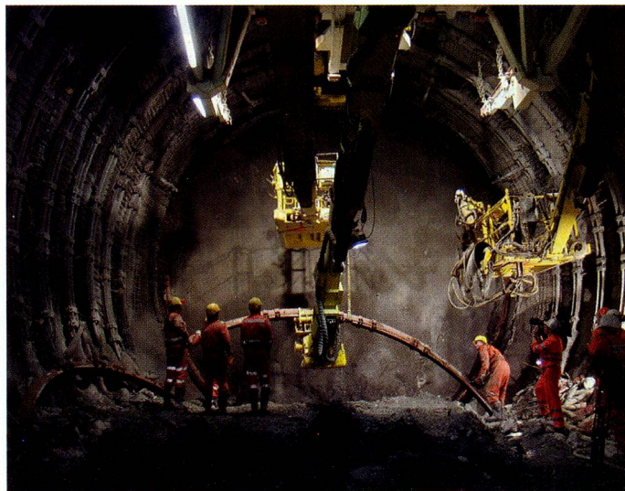
... to make the first breakthrough on 6 September 2006.
