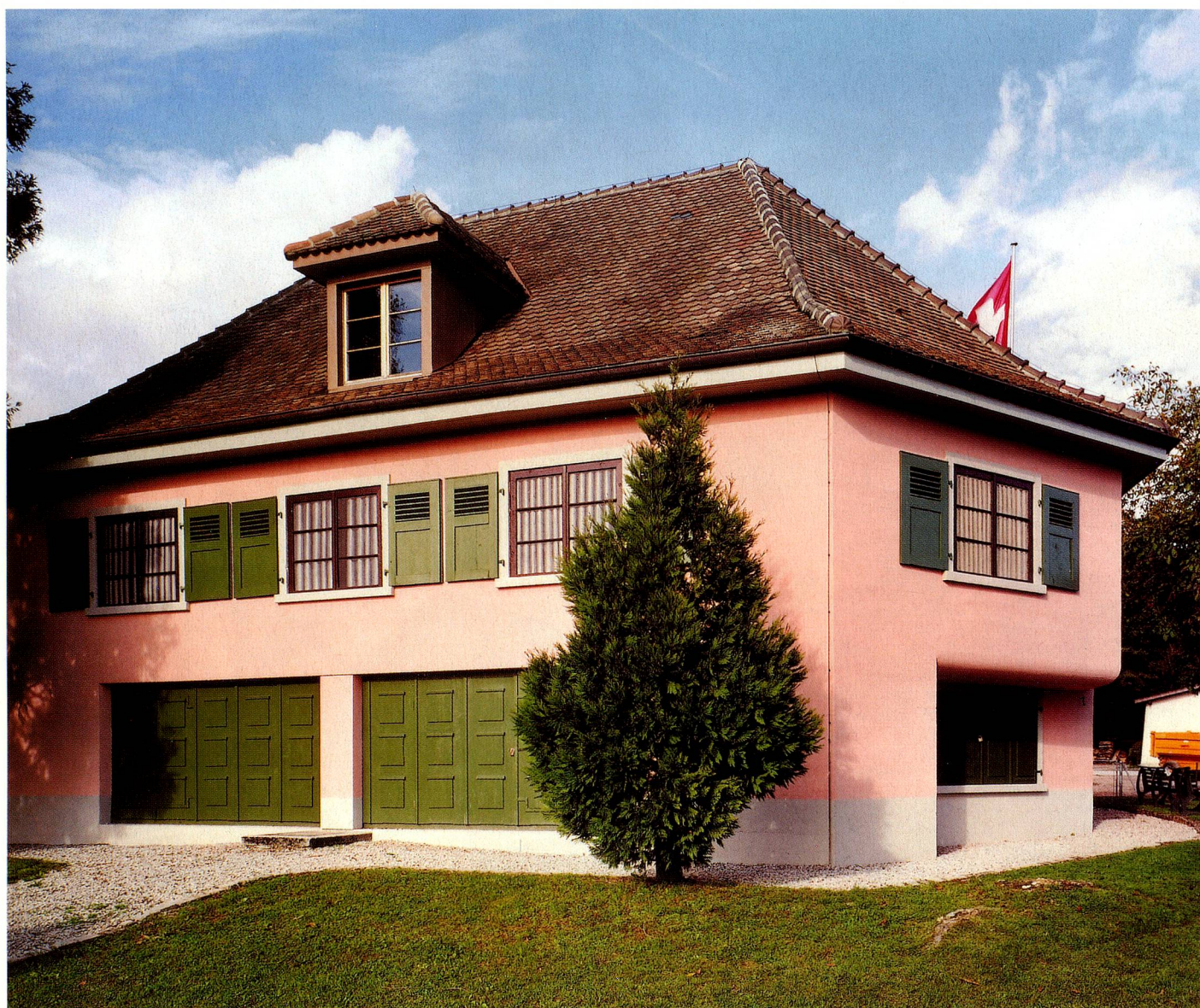
Villa, 1940, infantry bunker, Gland VD: solid construction with tiled hip roof and dormer window. Behind the template windows, curtains are painted directly onto concrete. The bunker is now used as a museum.
