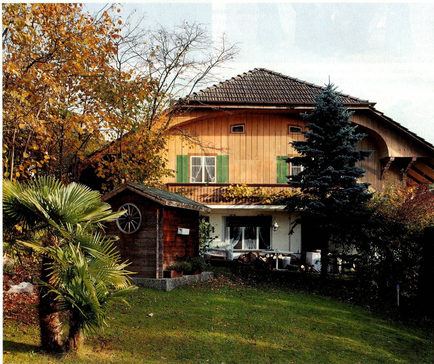
Chalet, 1941, infantry bunker, Hilterfingen BE: concrete building with tiled saddle roof and overhang. Windows, shutters and balcony balustrade are painted on wood cladding. Under the balcony is the bunker entrance, disguised as a window with the roller blinds half-closed.
