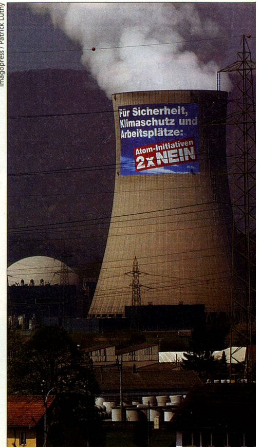
Voting slogans on the cooling tower of the Gösgen-Däniken nuclear power plant. The giant poster measures 64 x 44 metres.
