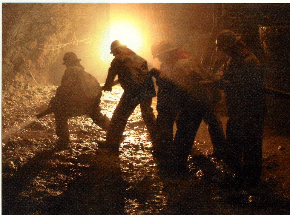
Teamwork is a must for underground construction.
