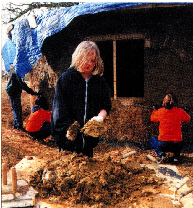
Students at work constructing a mud-and-straw building on the Pestalozzi estate in Sussex – helping them to have a greater understanding of sustainable development possibilities
