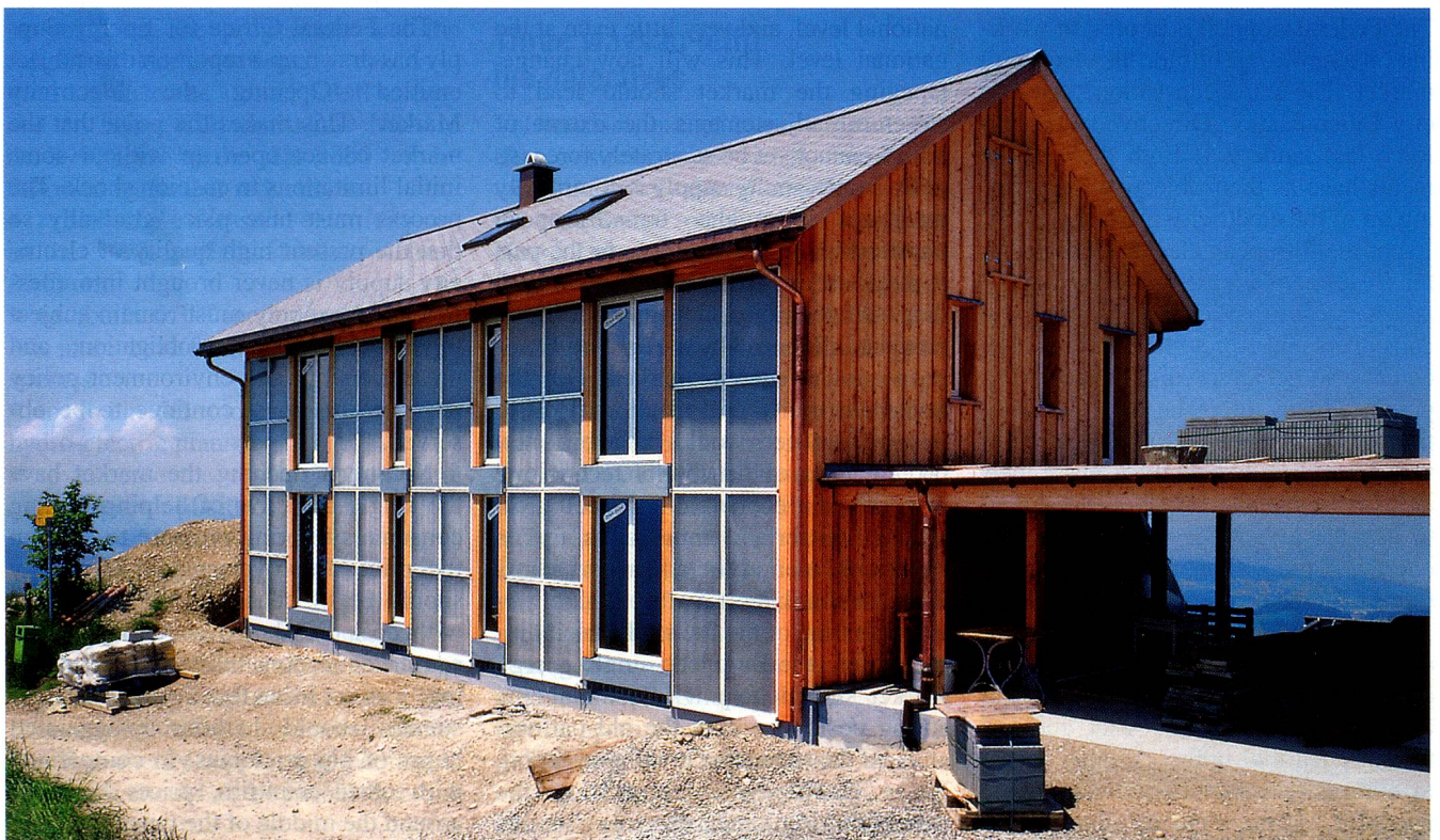
A pilot project in Canton Appenzell: the new technology of transparent heat insulation turns house walls into suppliers of solar energy. (Photo: Oerlikon Journalisten)
