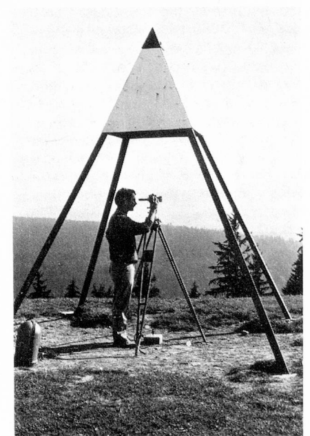
Measuring vertical angles with a theodolite
