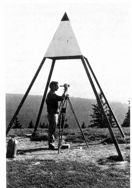
Measuring vertical angles with a theodolite
