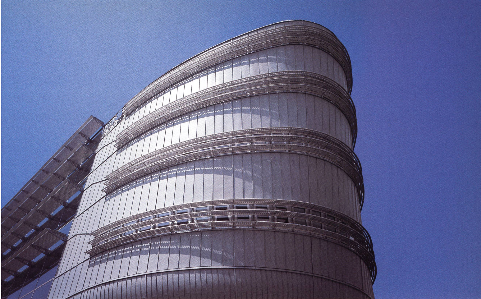
University of Surrey - Eihms Building - European Institut of Health & Medical Sciences, GB-Guildford; Architekt: Nicholas Grimshaw & Partners LTD, GB-London
