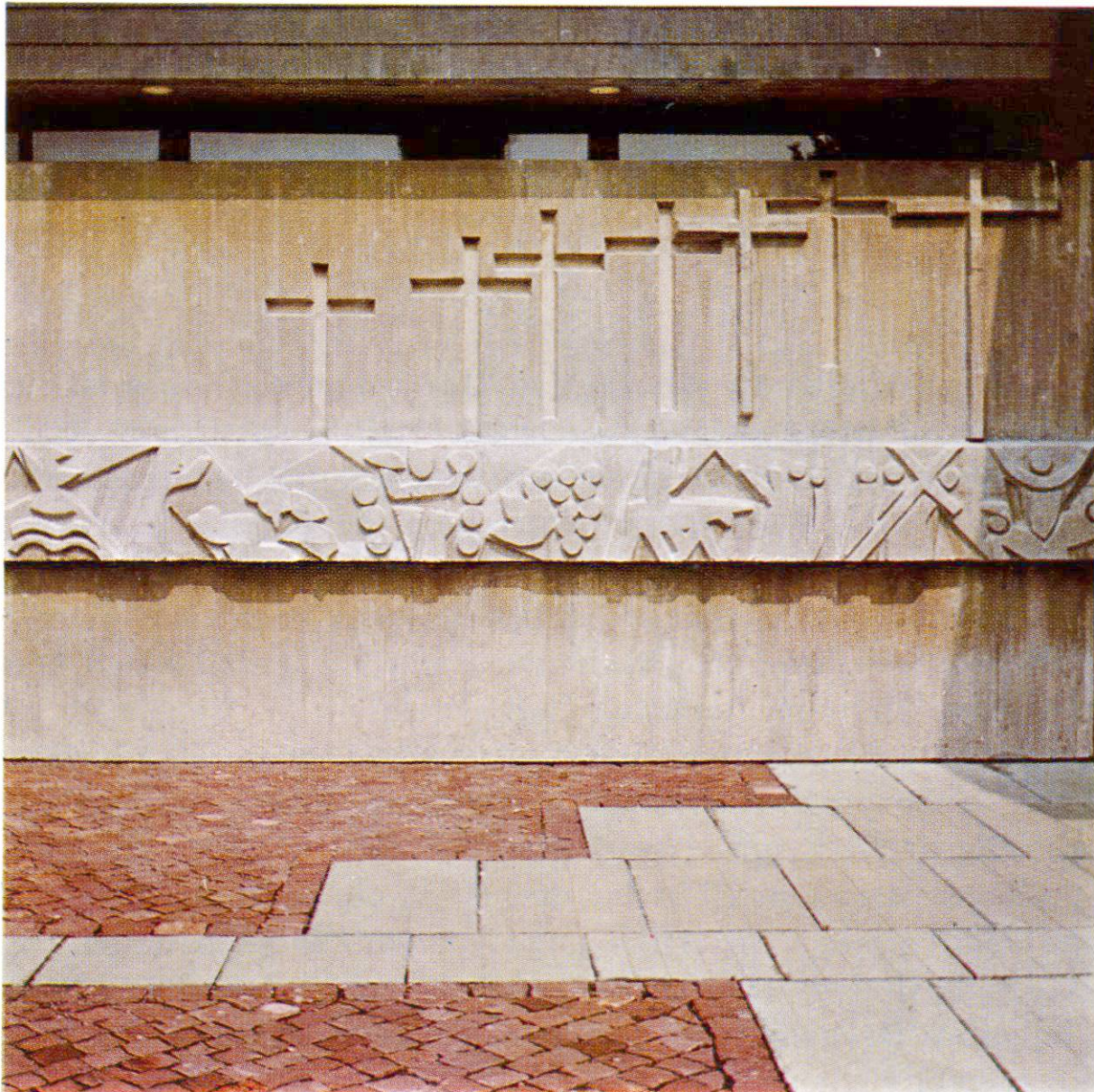
Detail des Beton-Reliefs
