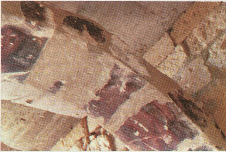
1. Mamshit, staircase hall, supporting arch
