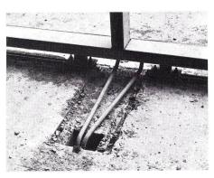
5 Elektrokanal / Chemin de cables / Cable duct
