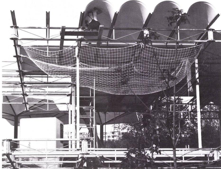
These structures, which are inhabited, were planned by the designers with a view to obtaining new findings; they were erected from the autumn of 1976 to 1977 in stages on a refuse dump, which had been closed for eight years. There are tested in the first instance wall elements of fibre-glass-reinforced plastic, which are also intended to be suitable for floor structures as well.
