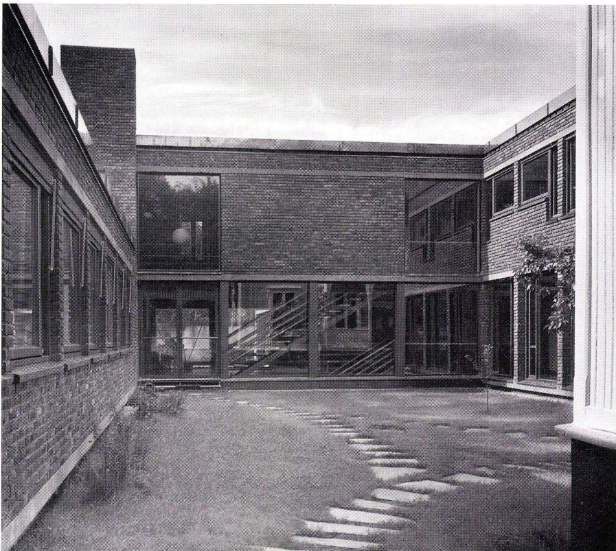
2 Innenhof. Cour. Inner court.
