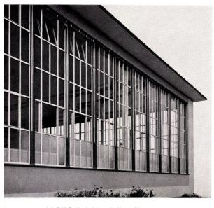
ALSEC-Leichtmetallprofile  $\mbox{K} = \mbox{2,25} - \mbox{2,5} \\ \mbox{Isolierglas-Elemente} \mbox{ K} = \mbox{2,5} - \mbox{3,0} \\ \label{eq:K}$
