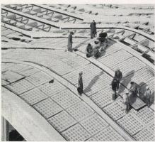
pression. Ferro-concrete frame on pendulum supports with horizontal wind bracings. Glass concrete as roof covering, closure of entrance hall in steel and glass between supports.
