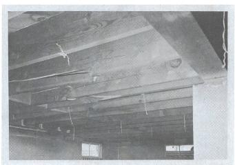
Figure 5.27. First floor joists of strengthened wood-frame house after a nuclear explosion (2.6 psi overpressure).
