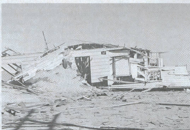
Figure 5.35. Rambler-type house after a nuclear explosion (5 psi overpressure).
