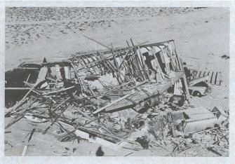
Figure 5.14. Wood-frame house after a nuclear explosion (5 psi overpressure).
