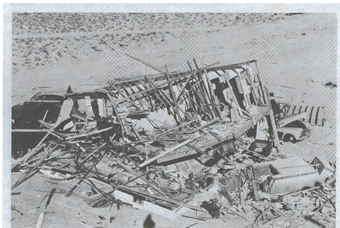
Figure 5.14. Wood-frame house after a nuclear explosion (5 psi overpressure).
