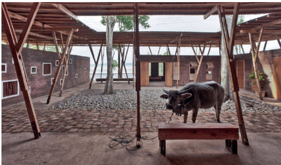
Vues du Cassia Coop Training Centre (Photos Pasi Aalto)
