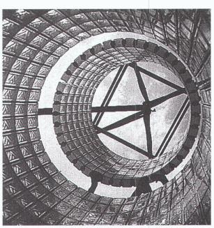
BRIQUES DE VERRE PRÉFABRICATION MAÇONNAGE SUR CHANTIER
