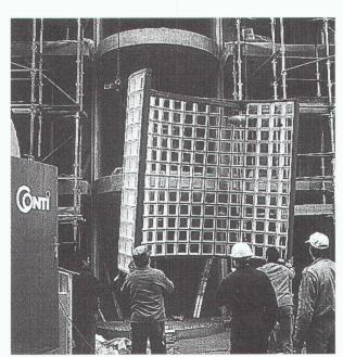
BRIQUES DE VERRE PRÉFABRICATION MAÇONNAGE SUR CHANTIER
